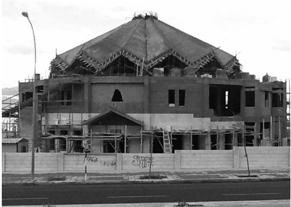
The construction work for the Church of Stella Maris in Aqaba as it was at the end of March.
